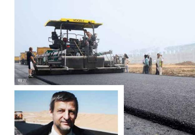
01 // The final touches: the surface course is made from a special asphalt containing aggregate with high resistance to polishing. This ensures that the road's good grip is maintained in the long term. The surface course was paved with an AB 600 Extending Screed in TV version.
